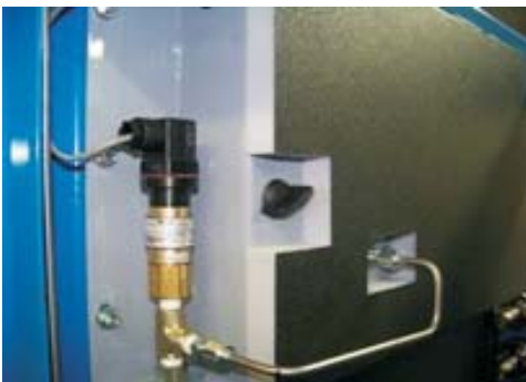
fig. 7.2-1 BAM interior view
